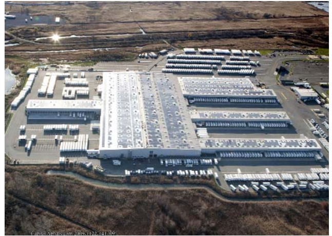
The FedEx Ground Woodbridge facility after panel installation. The facility has 538,000 square feet of roof space and fifty percent of the roof area was used for the solar panels and raceway.
