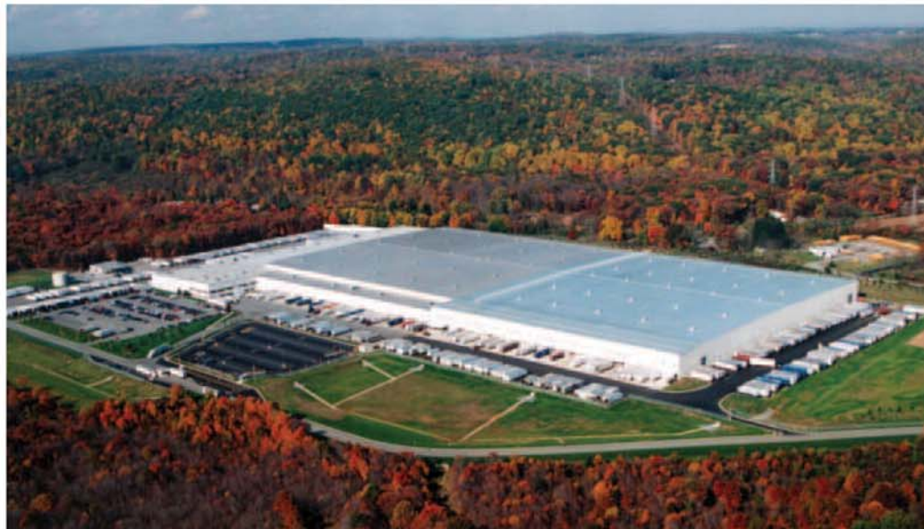
Toys “R” Us doubled the size of its distribution center in Mount Olive, N.J., with work completed in 107 days.
