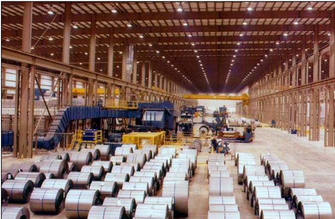
BES provided all erection and sheeting of this 770,000 square foot steel processing facility and was a major contributor to the project being completed 10 months early and under budget.
