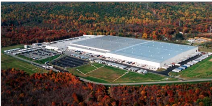
The 519,200 square foot expansion to this existing warehouse was erected and sheeted by BES in just 74 working days.
